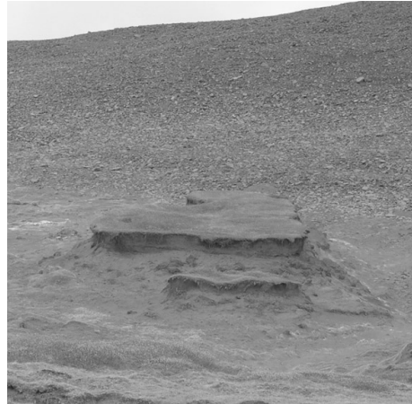
Figure 2 Massive erosive decay of soil body
